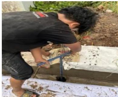
**Gambar 2.** Proses Boring tanah.
